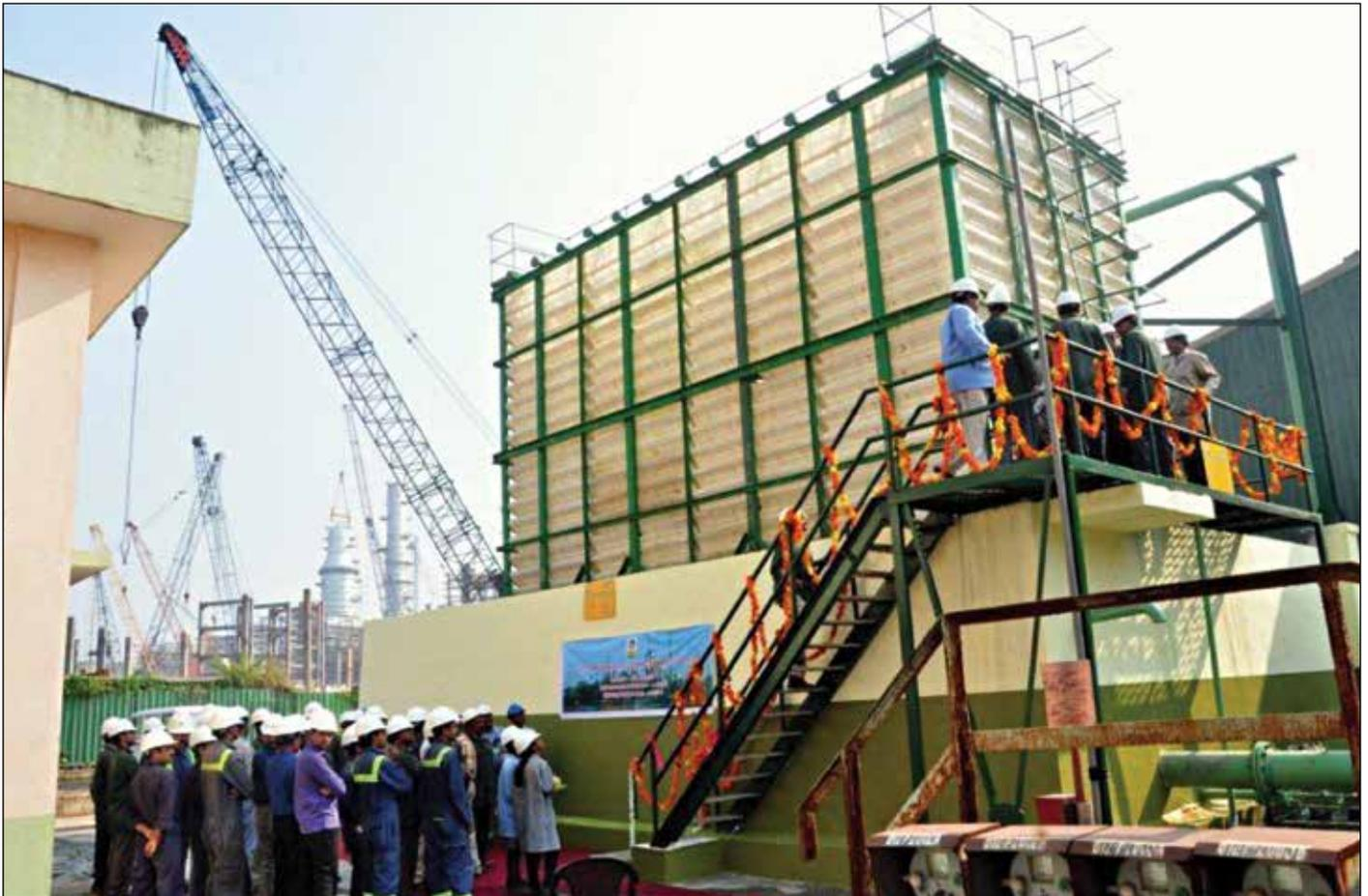
**Figure 2: Installation of Jet Cooling Towers at GT2 Power Plant, BPCL site.**
