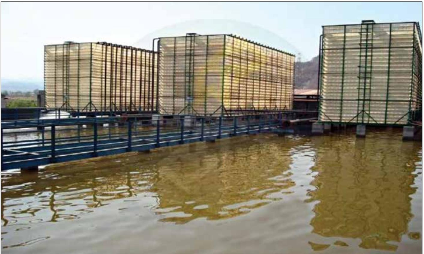
Figure 1: Jet-type fanless cooling towers
